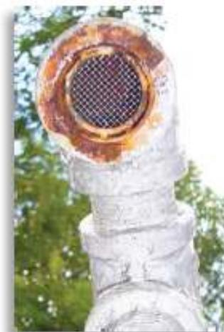
This wire mesh end-of-line flame arrestor is part of a pressure relief assembly on a liquefied petroleum gas transfer apparatus.
