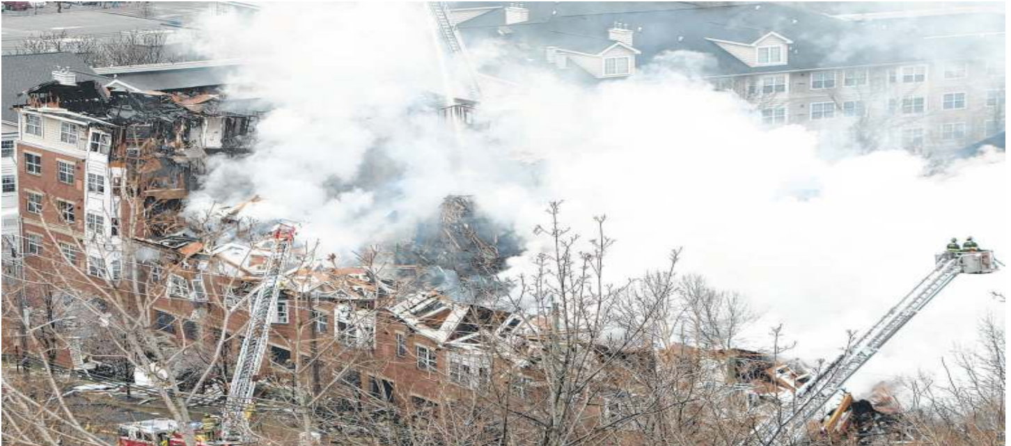
Smoke continues to rise from the Avalon at Edgewater apartments on Thursday, a day after flames raced through the complex. (PHOTOS BY S.P. SULLIVAN/NJ ADVANCE MEDIA FOR THE STAR-LEDGER)
