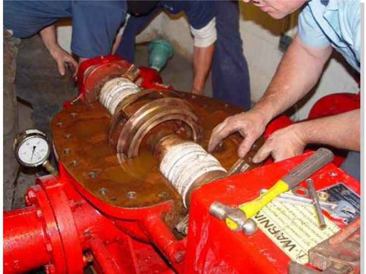
A fire pump service technician inspects the exposed vane for evidence of cavitation. (Photo courtesy of Keith Heckler, Rockville Fire Department, Maryland)
