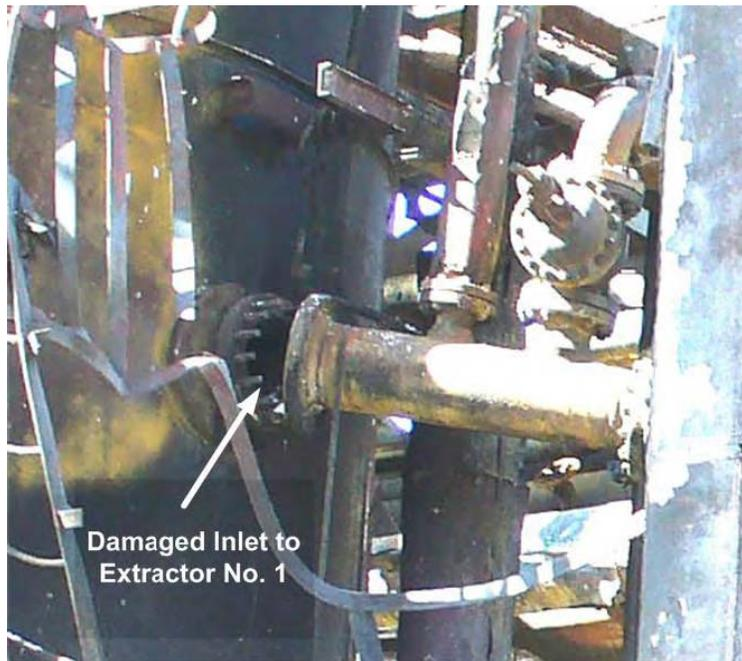
Figure 8. Damaged 10” propane inlet on Extractor No. 1
