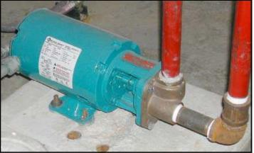
3) The fire pump *start* point should be 5 psi (0.34 bar) less than the jockey pump *start* point. When additional fire pumps are installed in series, use 10 psi (0.68 bar) increments for each additional pump.
